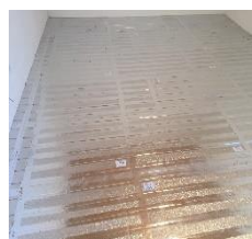
The room after installation and adhering the cables with metallic tape
