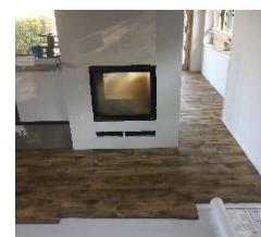
Floating floor laying on the insulation boards + Line™T10 + impact insulation
