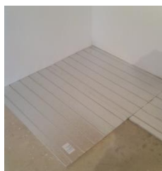
Gluing AL IzoLine20™ to the floor
