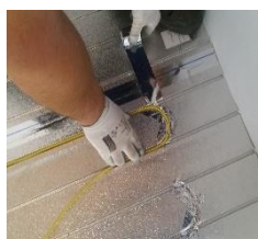
Fixing the boards together and adhering the cables Line™T10.
