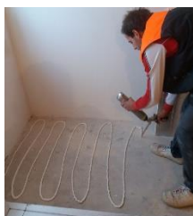
Spray application of the polyurethane adhesive
